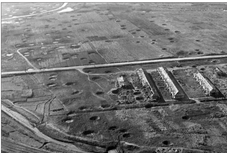
Fig. 3. Bomb craters around Hŭngnam Industrial Complex, North Korea, 6 November 1950. Note the many bomb craters on the broad field surrounding the buildings that were targeted in this attack. (Credit: National Archives and Records Administration)
